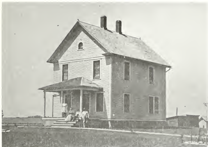
Overseer's house at Mile 26 from the Illinois River north of Sheffield. (Photograph courtesy of Hennepin Canal Parkway.)
